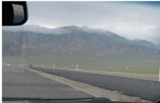
KHARGOS- LIYUNGANG HIGHWAY (NEAR SALYMOON LAKE, XINJIANG) UNDER CONSTANT REPAIR
