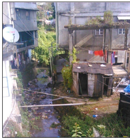
Plate3: Picture of buildings with poor sanitary conditions at a site in Laban, polluting Umshyrpi River.
