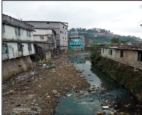
Plate1: encroachment of buildings into Umkhrah River at a site near Demseiniong.
